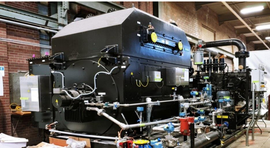
NEW TURBINE GENERATORS 7 and 8
