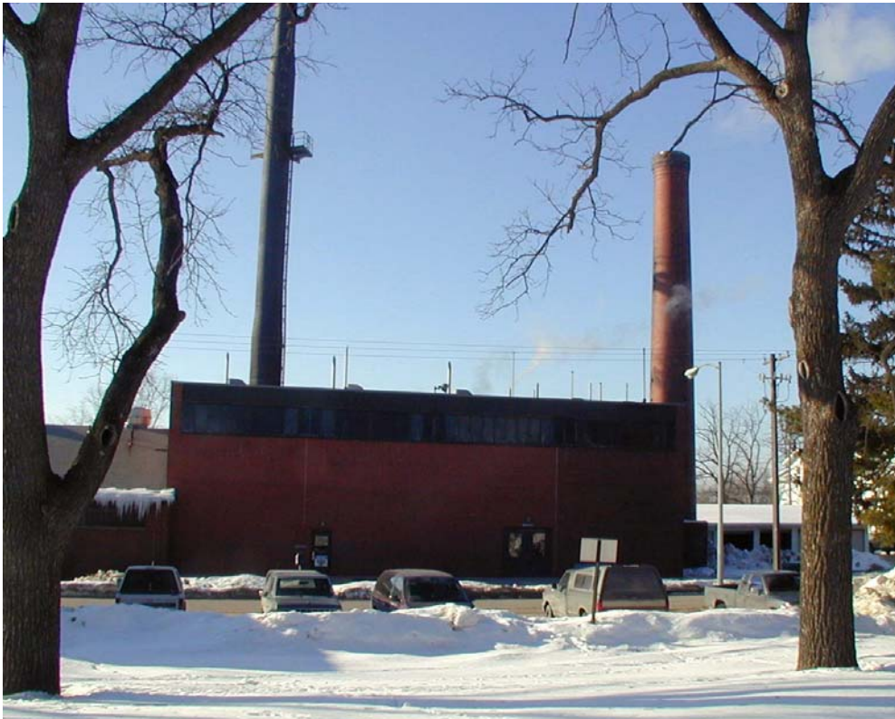
Power Plant at Oakdale
