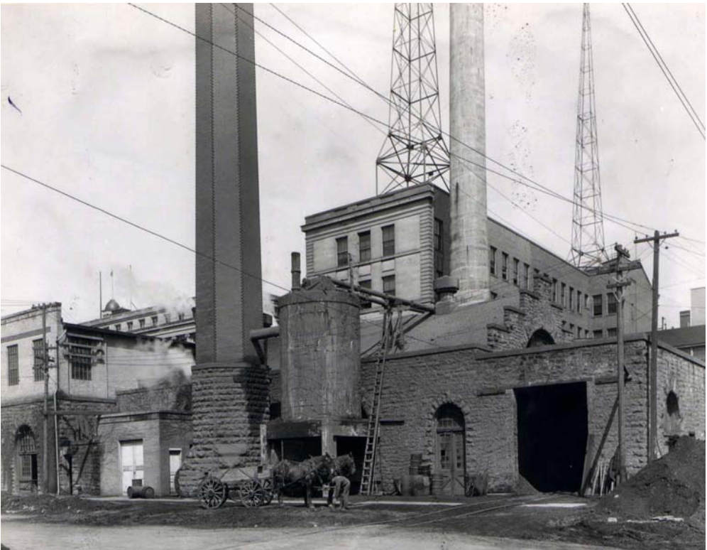
Old Power Plant on Madison and Washington
