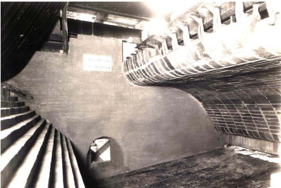
Interior of an original coal boiler
