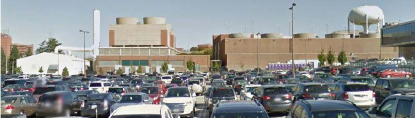
EXISTING GROUND VIEW FROM KINNICK PARKING LOT
