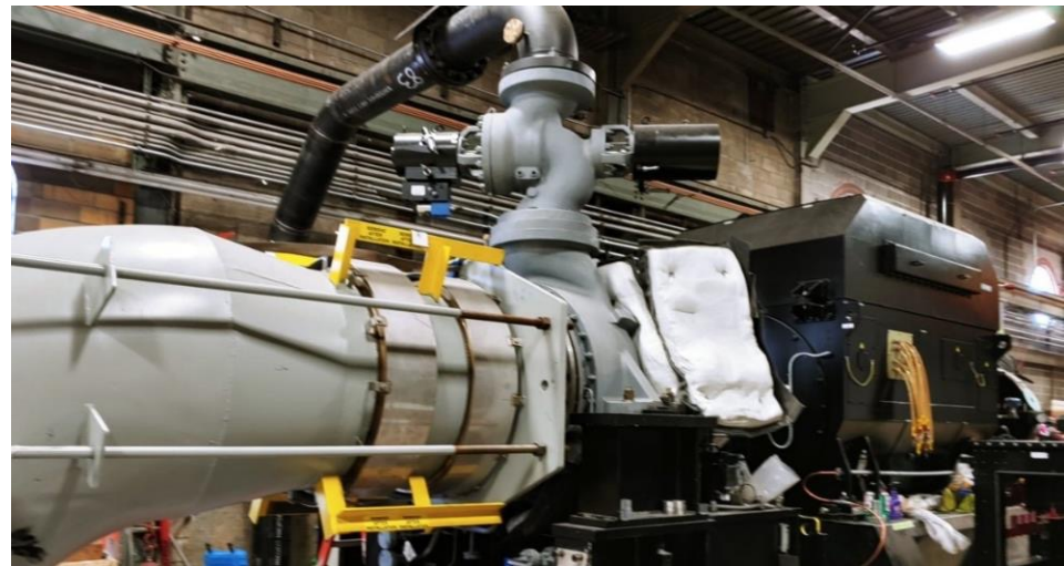
NEW TURBINE GENERATORS 7 and 8
